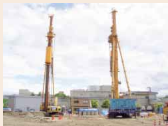
Cleanup work (NEC Yamagata's former Takahata Plant)
