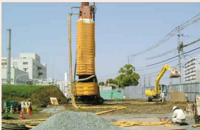
Soil cleanup was completed in April 2006.
